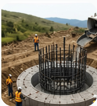
3 Foundations excavation and reinforced concrete foundation
