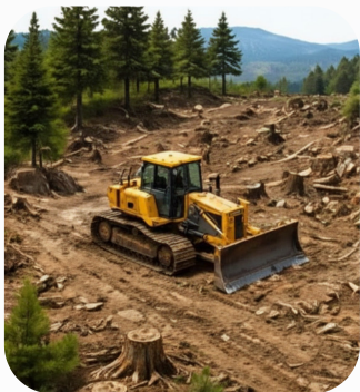
1 Site preparation and vegetation clearance
