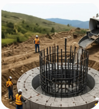
3 Foundations excavation and reinforced concrete foundation
